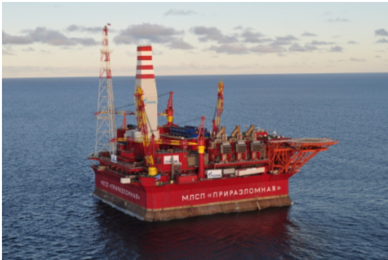
▲ Figure 1. Here is a photo of the rig Prirazlomnaya.
